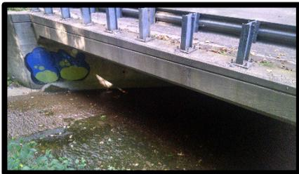
**[BMS 08-7238-0596-0006]** Glen Road (T-596) over Pond Hill Run: This structure is located on Glen Road off of S.R. 187 North. The structure is a concrete culvert, built in 1994, with a span length of 26 feet and a width of 24.2 feet. The last inspection report dated July 22, 2015 indicates the overall condition of the structure as good. The structure has no posting restrictions and is inspected on a two year (24 month) frequency.
